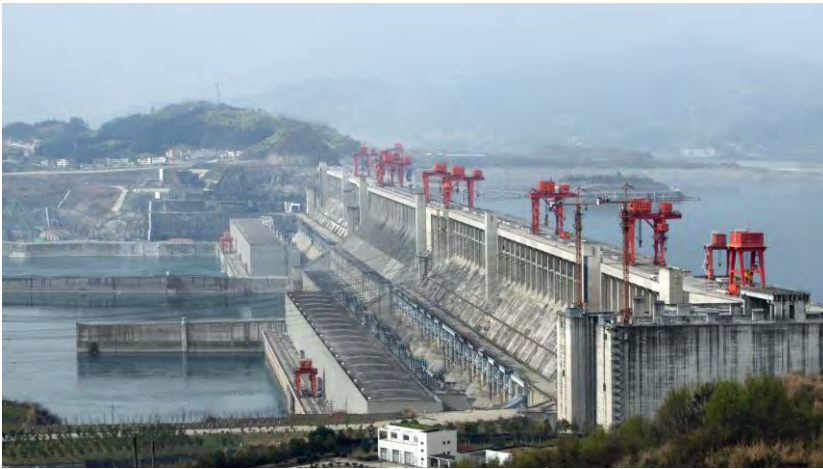
Fig. 1 – The Three Gorges Dam, China
